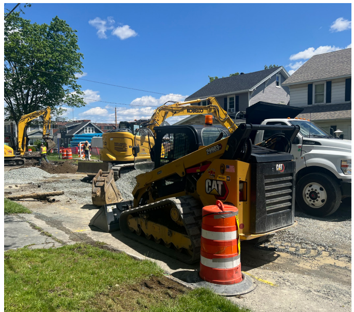
The South End Infrastructure Upgrade Project continues work on Hutton Street
