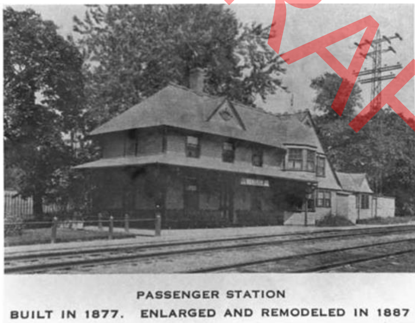
Figure 4 Menands Passenger Station (no longer standing)
