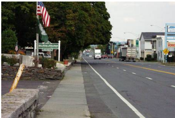
Above: Residential scale between Rt. 378 & Brookside Ave
