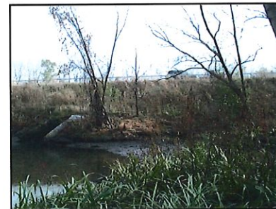
Culvert under I-787
